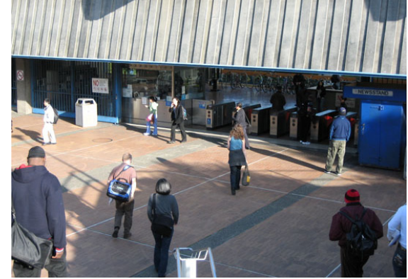
Glen Park BART Station
